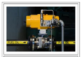
Emergency isolation valve with local (thermal) and remote shutoff. (Photo courtesy of Assured Automation)
